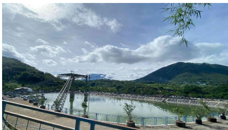
Figure 6.23 Water Reservoir Application
