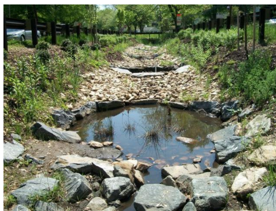
Figure 6.10 Loose Stone Check Dam
