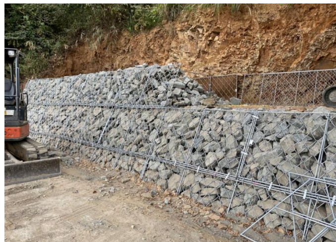
Figure 6.11 Gabion Check Dam
